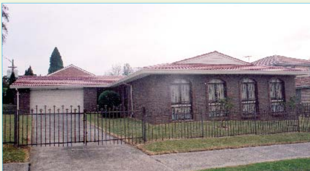
Lixouri House North Ryde
